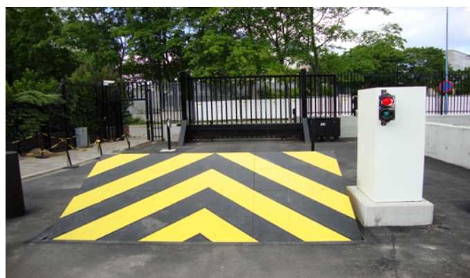
Terra Blockers control cabinet installed next to blocker
