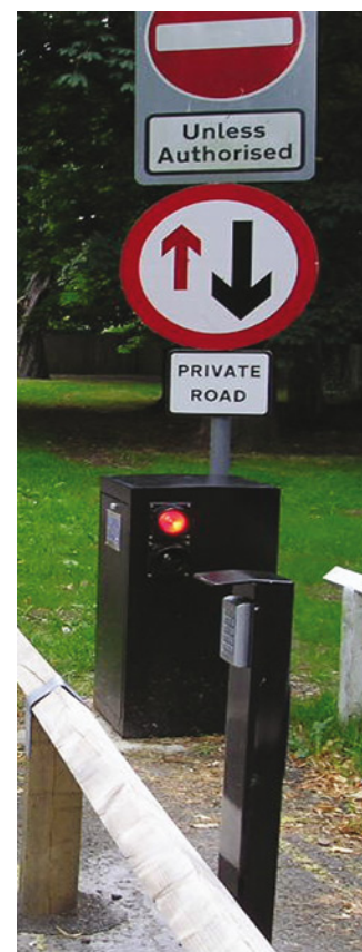
Terra Blockers control cabinet installed next to blocker
